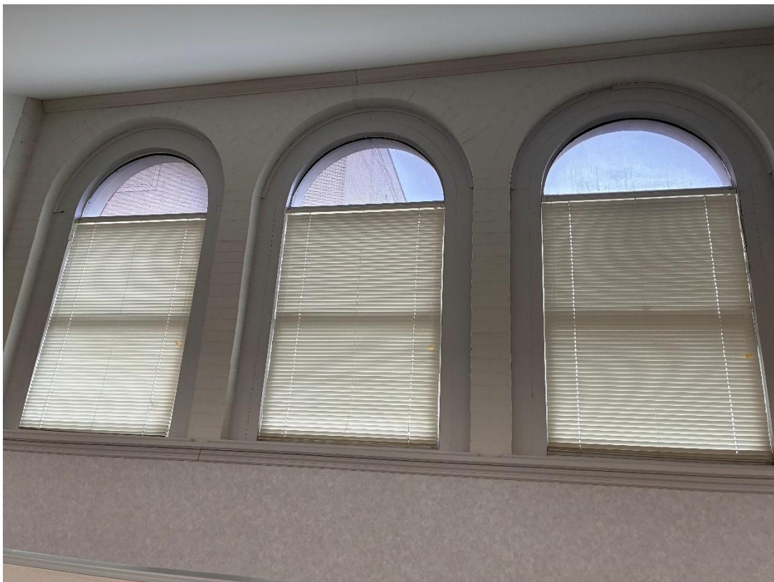
4 th Floor Office Space
