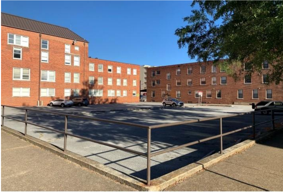
Subject Surface Parking Lot
